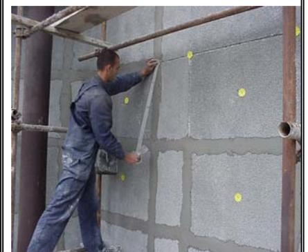
Application of Simplolit plates in upper floors and attics construction is also very practical. Namely, these plates can be used as both thermo-insulation and suspended ceiling plates, which could be just skimmed with cement paste mixed with fine sand, or with cement-based glue right after mounting. Upon request, they may also be plastered using a thin (3-5 mm) layer of cement-lime plaster, or just primed and painted.
